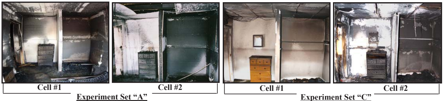
Figure 32-35 – North Wall (left to right) Exp. Set “A”: Cell #1, Cell #2; Exp. Set “C”: Cell #1, Cell #2
